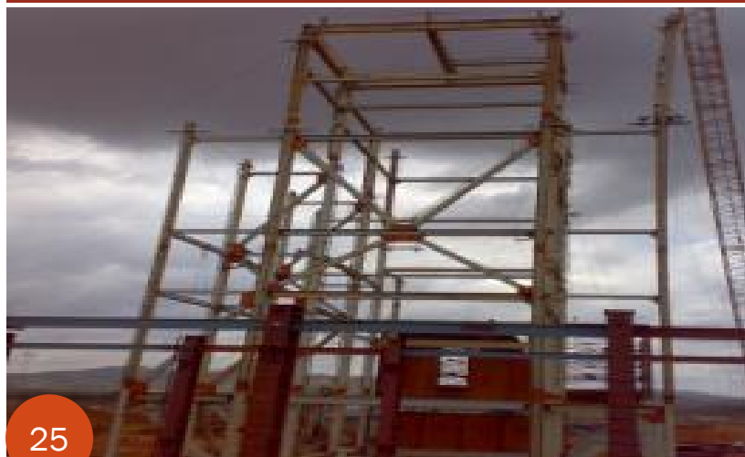
BTG Package:Boiler#1: 4 Tier column erection.
