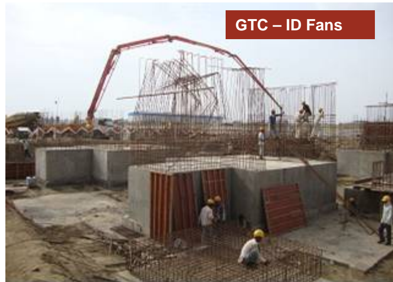
Shuttering work for TG#1
