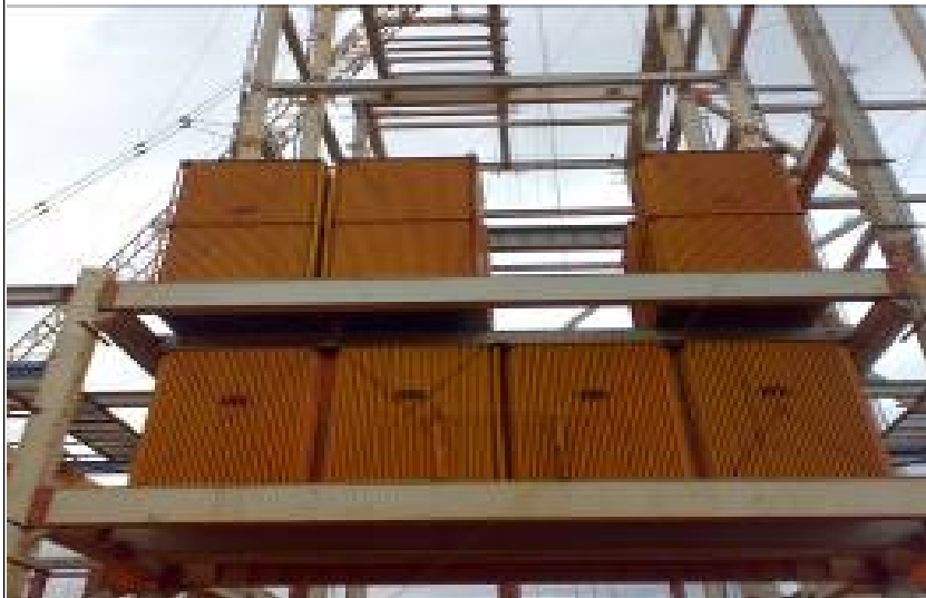
BTG Package:Boiler#1: 4 Tier column erection.
