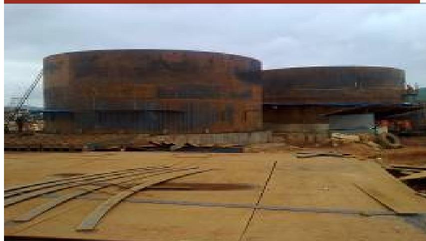
Calcination Area: Stack #1: 4th shell completed
