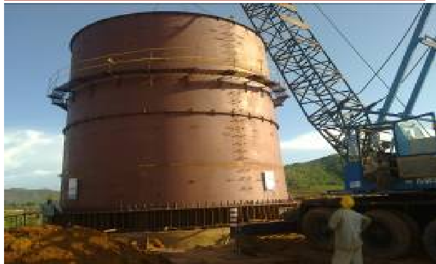
Calcination Area: Stack #1: 4th shell completed
